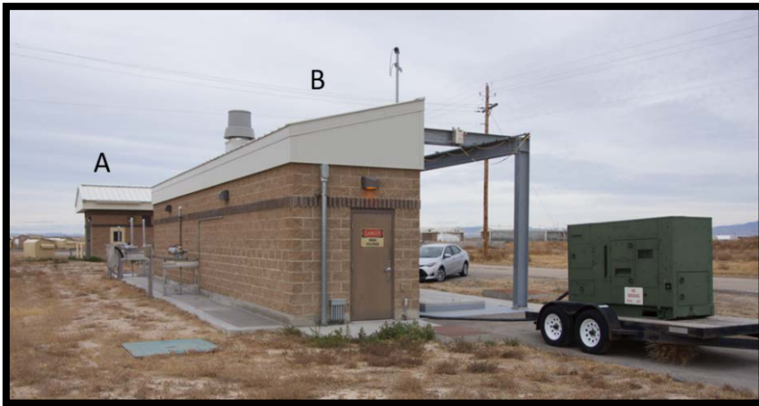
MHAFB headworks buildings—inlet & grate (A), grinder & pumping station (B)
